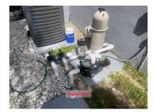
Epoxy was applied as a temporary patch to the leaking area(s) so that it can be ensured all leaks have been identified and all appropriate repairs have been quoted.
