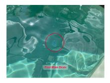
Found leak around pop up body. Patched with epoxy. Recommend proper repair.
