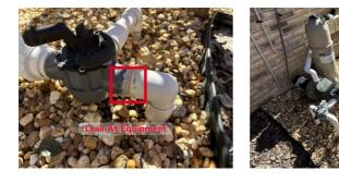
Air is leaking around the: Jandy/ball/gate valve Additional Notes: N/A
