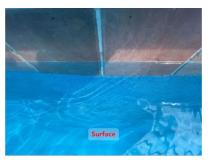
Epoxy was applied as a temporary patch to the leaking area(s) so that it can be ensured all leaks have been identified and all appropriate repairs have been quoted.
