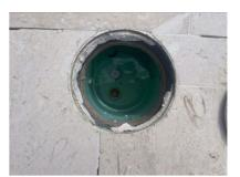
Found leak around overflow line. Patched with epoxy. Plugged overflow line as requested, as it sits too low in the pool.
